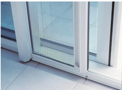
This system is the most commonly used one. It can be utilised with face fit (flush), with angles or with our standard range of treads, either raised section or flush floor situations where extra support is required. The standard track is 25 mm high and 20 mm wide so if flush-fit is desired for the double French door situation, allowance for the track is required.
